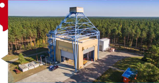
Technical Safety Test Site, Horstwalde
