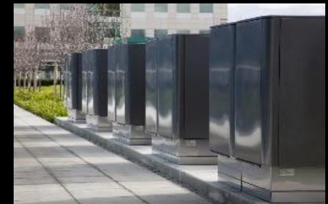
BLOOMENERGY Sc-SOFCs deployed at NASA building
